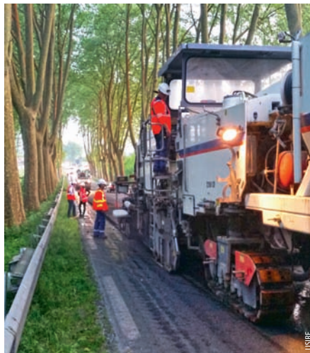
Photo 2 Final part: Application of the cold asphalt concrete
