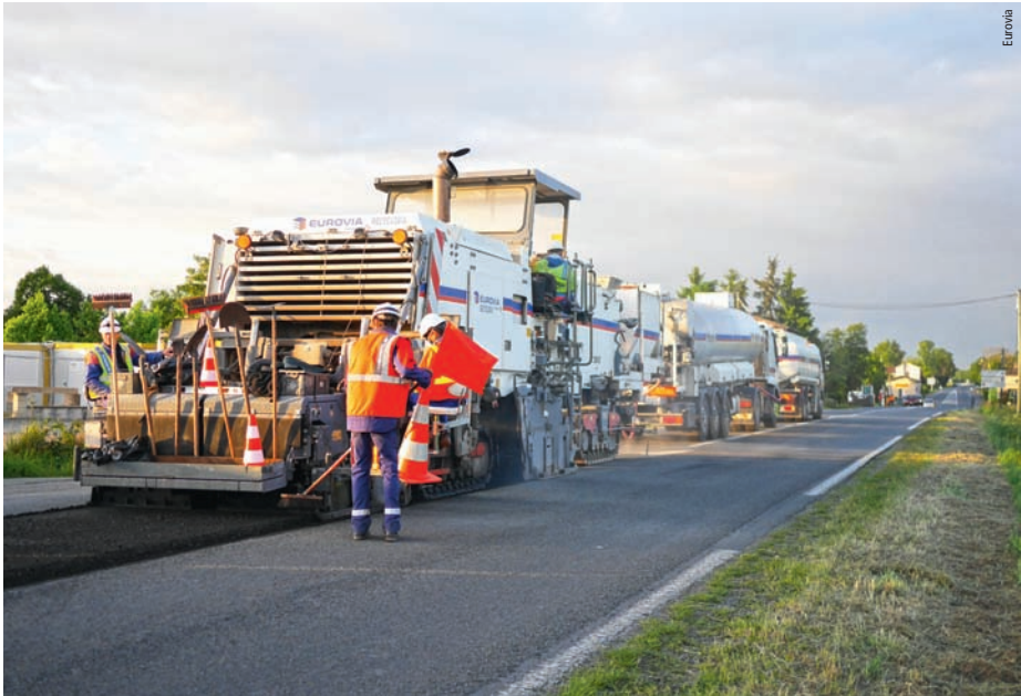
Cold in place recycling machinery
