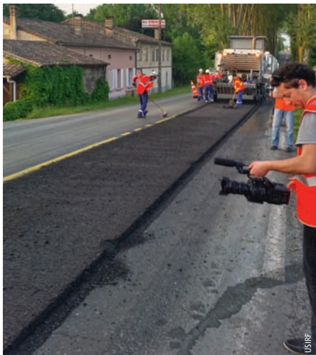
Photo 1 Cold in place recycling
